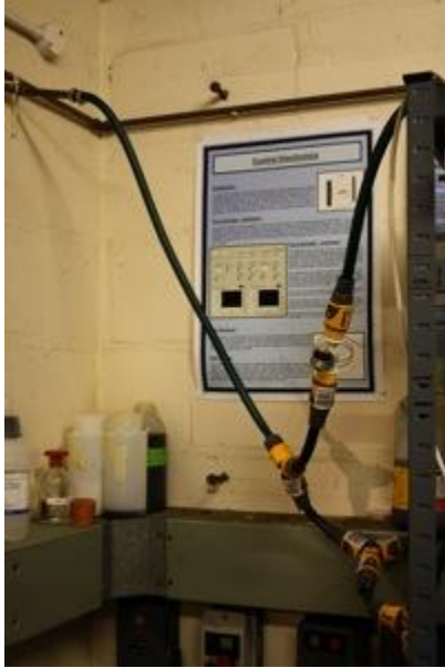
Figure 10.12: Mains Water Supply Connections.
